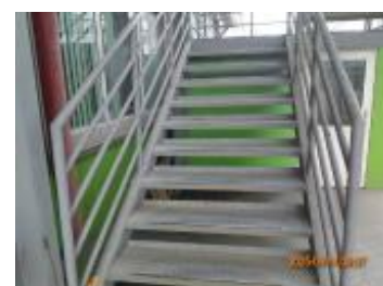
35. Stairwell equipped with both handrails.jpg
