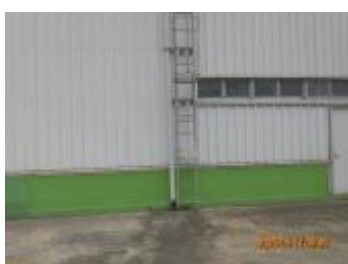
37. Vertical ladder equipped with safety cover.jpg
