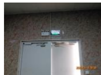
19. Emergency exit equipped with exit sign and emergency light.jpg
