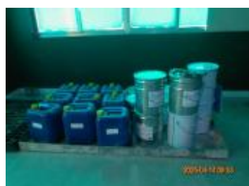
24. Chemical containers were stored in secondary containment at the chemical storage area.jpg
